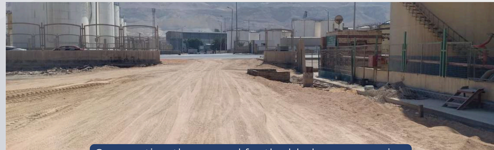
Compacting the ground for the blade manouvering
