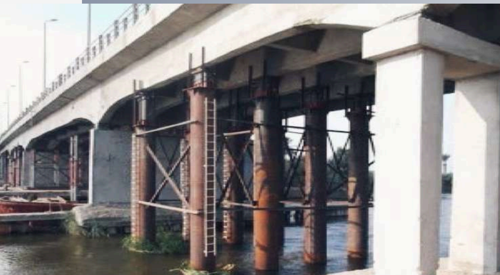
Enforcing Banha's bridge to bear up to 300T instead of up to 90T
