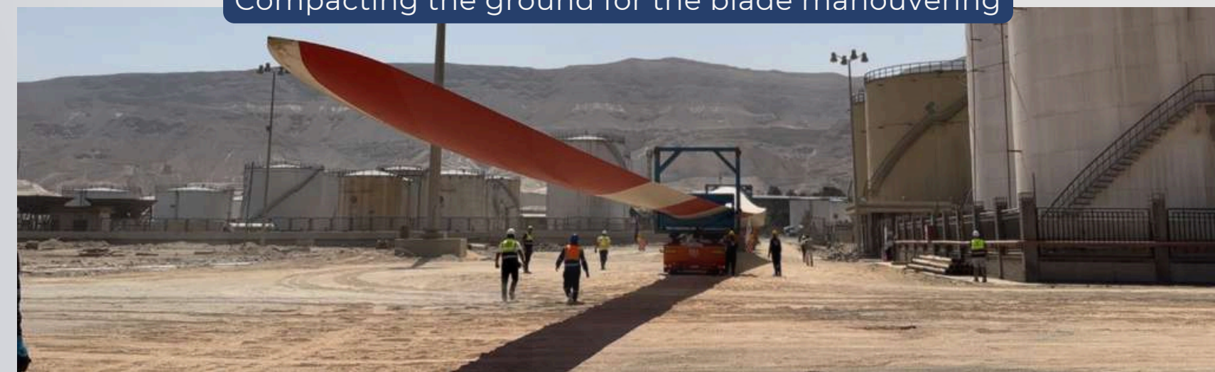
Compacting the ground for the blade manouvering
